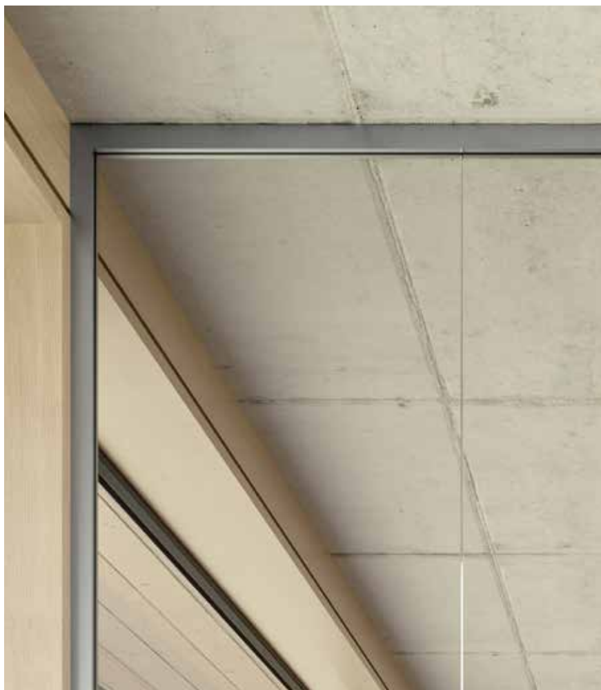
◀ Connecting to wall, ceiling or floor A perfectly fitted border all round: The wall connecting profile provides a secure hold for the glass.
